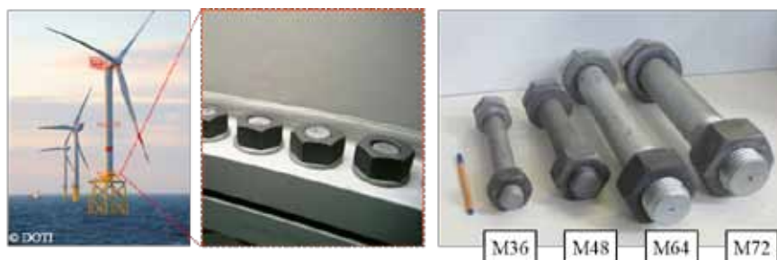
Figure 24: Positions of ring flange connections in a support structure with jacket supporting structure (left) and HV bolt sets with large diameters (right)
