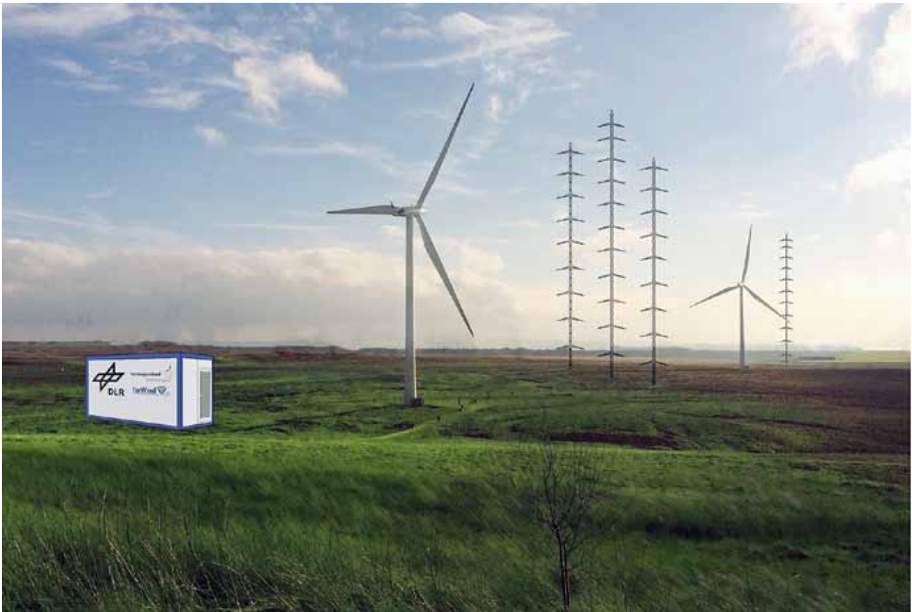
Figure 1: DFWind research wind farm consisting of two wind turbines of the current multi-MW class and meteorological measurement masts
