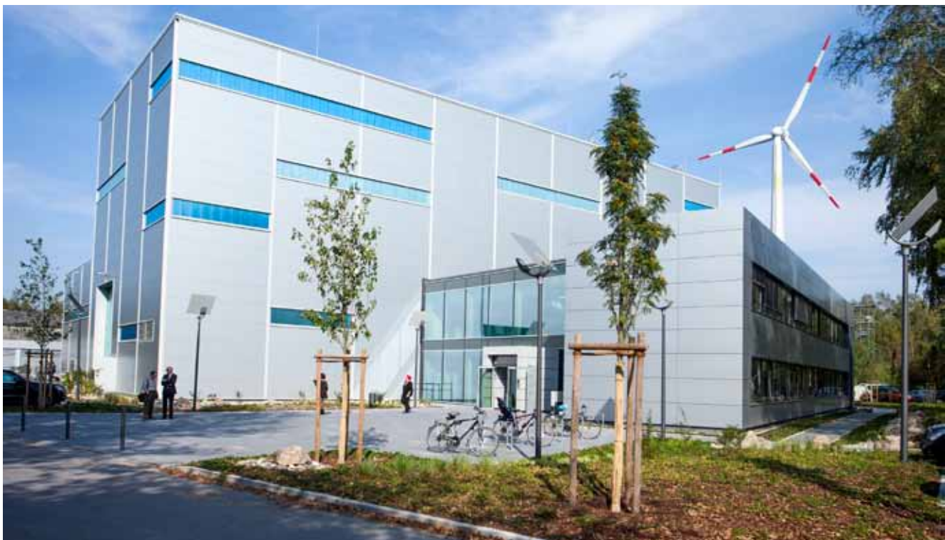
Test Centre for Support Structures (TTH) in Hannover-Marienwerder, picture: Mathias Schumacher, Leibniz Universität Hannover
