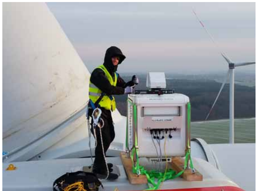
Figure 3: Installation of long-range LiDAR measurement system on nacelle of eno 114 wind turbine.
