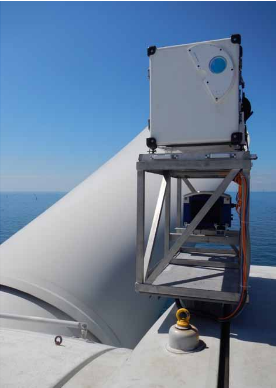
Figure 5: Mounting of Whirlwind 1 and a Leosphere WINDCUBE® lidar combined with the Stuttgart Wind Energy (SWE) Scanner from DEWI GmbH, Wilhelmshaven, on a wind turbine in alpha ventus , October 20th 2014.
