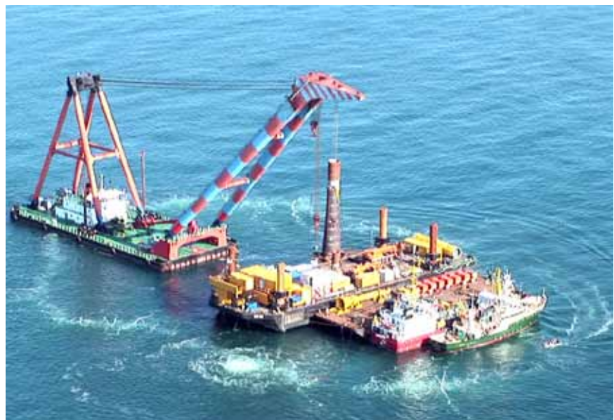
Figure 1: Big Bubble curtain installed at FINO3 construction site in 2008 [1]
